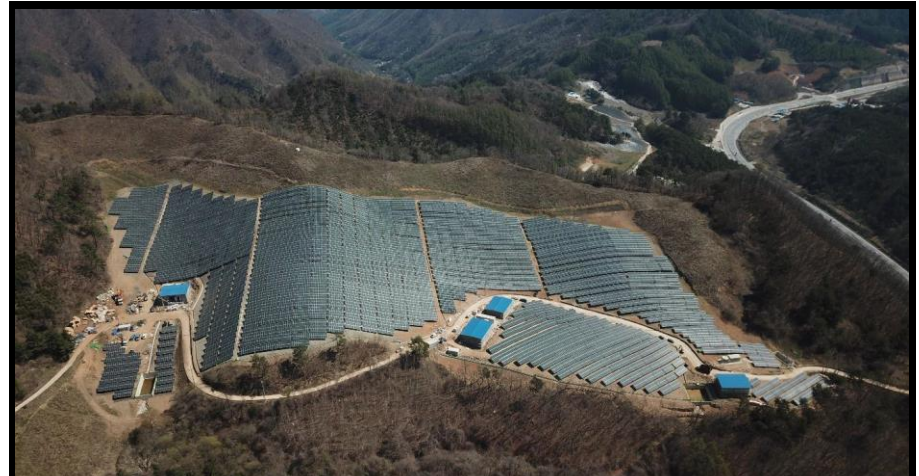
Jeongseon-gun Nexpo Solar Power Plant 8 MW solar power plant
