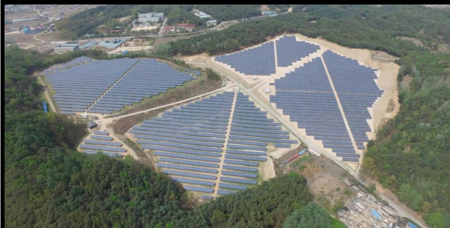
Chuncheon 10 MW solar power plant (2 x 3MW, 2 x 2MW)
