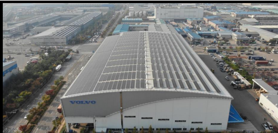
Solar Road No. 2 1.95 MW solar power facility
