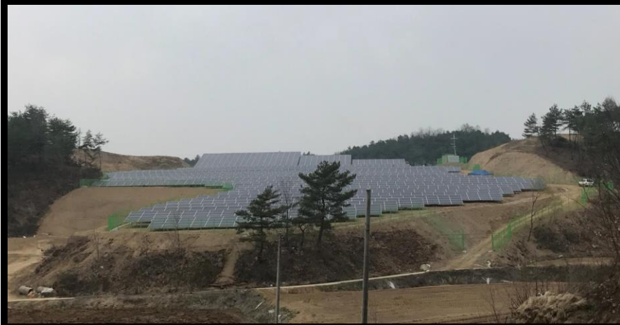
1.7 MW solar power plant in Yeongju
