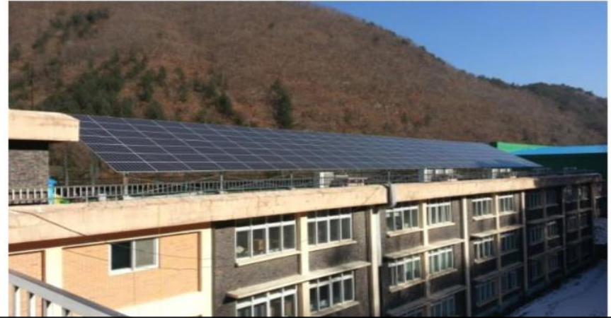
Gangwon Elementary School 51.94kW
