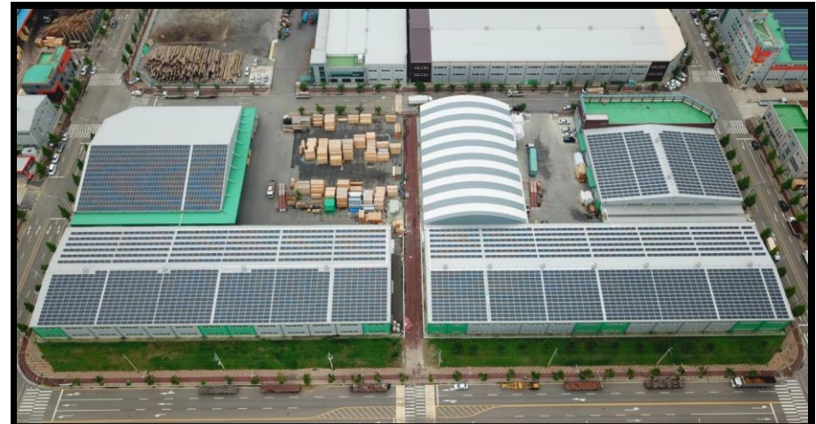
Incheon K-Won 1.24 MW solar power plant
